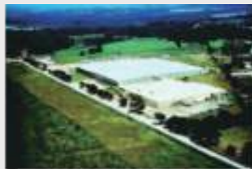
McQuay Auburn Factory, USA
